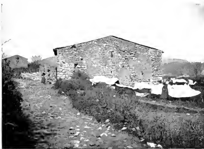
FIGURE 6. — VIA CIVITA, LOOKING NORTHWARD FROM 5
